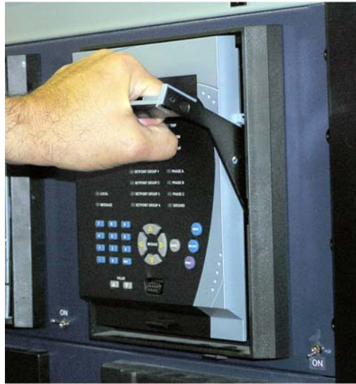
FIGURE 3-6: Rotate handle to stop position
