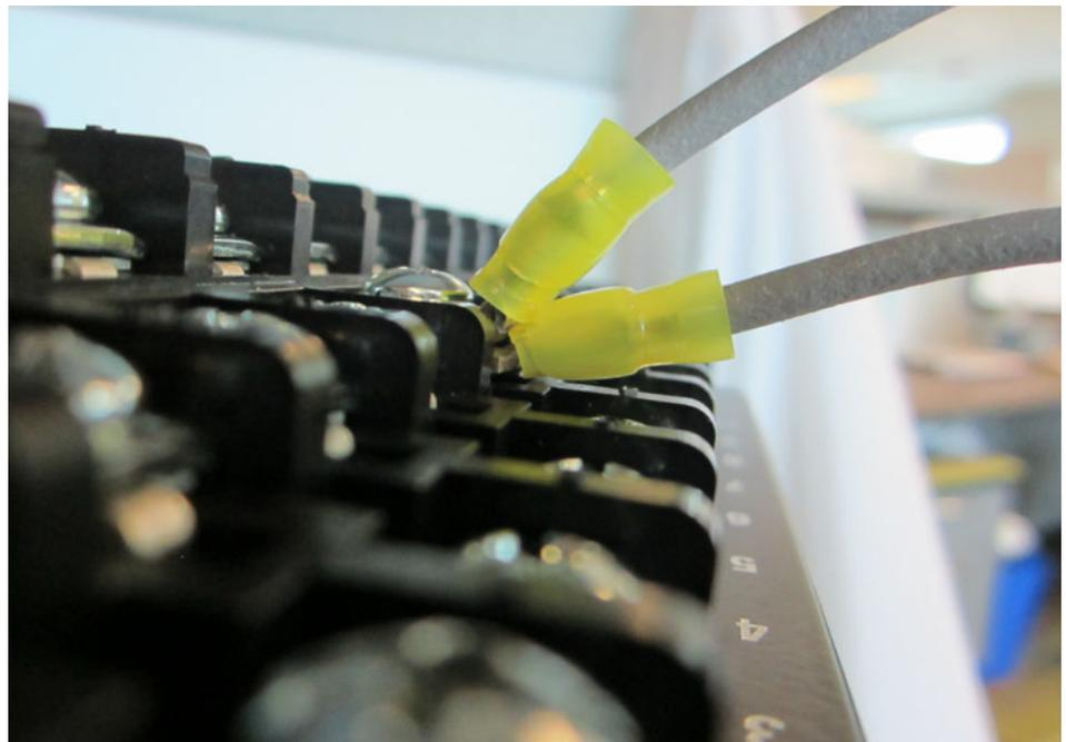
Figure 16: INCORRECT INSTALLATION METHOD (lower lug reversed)
