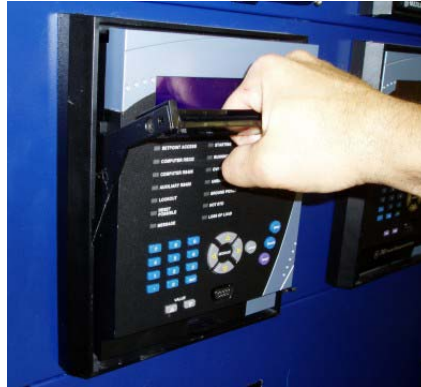
FIGURE 3-6: Rotate Handle to Stop Position
