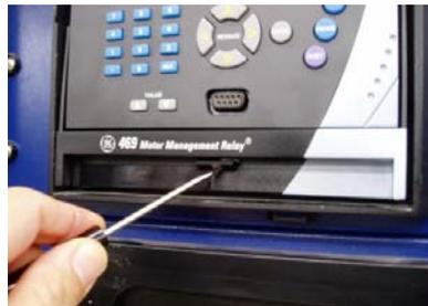
FIGURE 3-7: Press Latch to Disengage Handle
